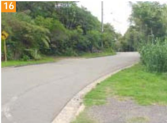
*A barrier kerb with a fully unsealed footway with vegetation occupying most of the space.*
