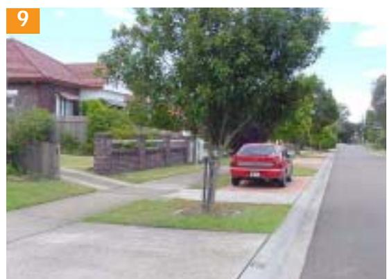
Footways may contain paved bays that are being used for parking. Photo 6 shows storage gaps where driveways are adjacent. Photos 7 to 9 show roll-top kerbs.
