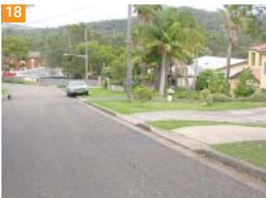
A barrier kerb with a wide fully unsealed footway except where there are driveways.
