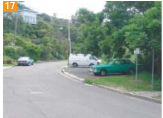
A barrier kerb with a fully unsealed footway except where there are driveways. Gardens also protrude onto the footway.
