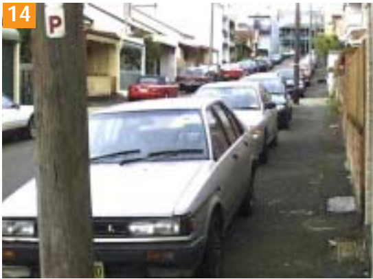
A barrier kerb with narrow fully sealed footway.
